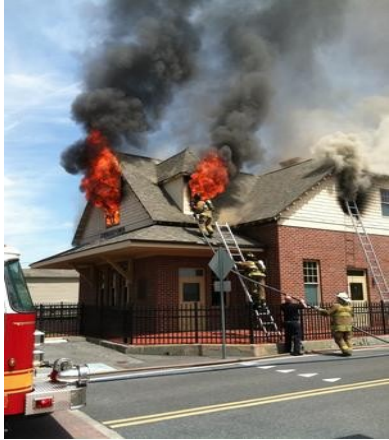
Georgetown Train Station Fire - 2012
